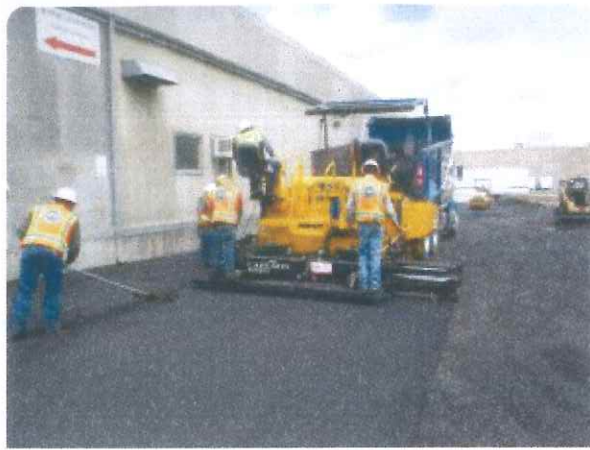
Leveling installed to promote drainage away from the building.
