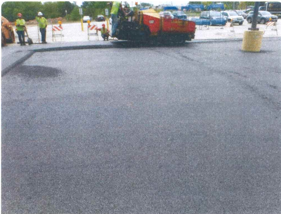
Correction of slope through the use of an asphalt leveling course.
